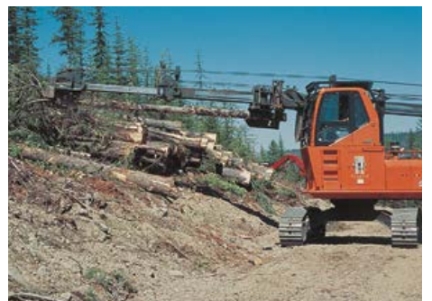
The stroke-boom delimeter operates at the landing or roadside, removing tree limbs and top, cutting the stem into logs and stacking them.
