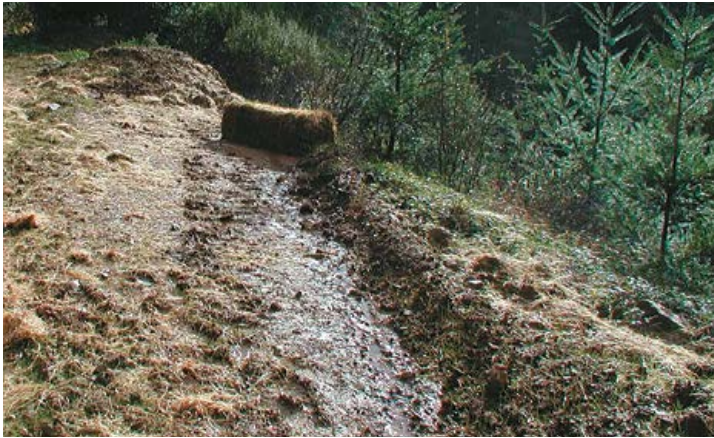
Hay bales or small slash windrows can reduce stream sedimentation. They slow surface water and trap sediment.
