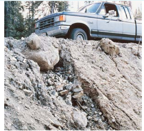
Soil sloughing off a road cut.
