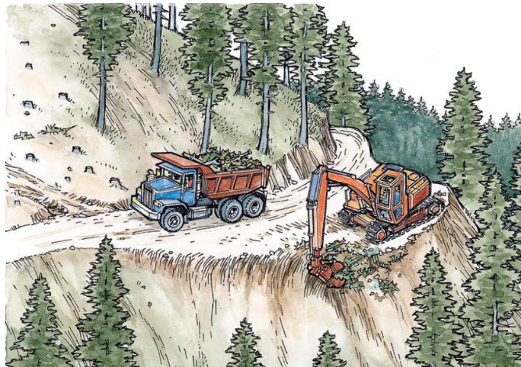
Remove excess material from landings and place it in stable locations.
