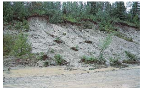
Poor road surface drainage caused this fill slope erosion.
