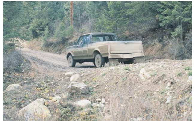
The drain dip bottom is sloped to carry water from the inside to the outside of the road surface, onto natural ground.
