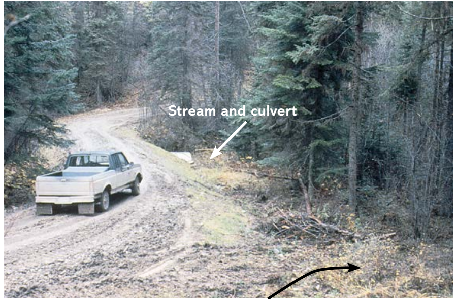
Route ditch drainage through a filter of vegetation and undisturbed soil so sediment can be removed before water reaches the stream.
