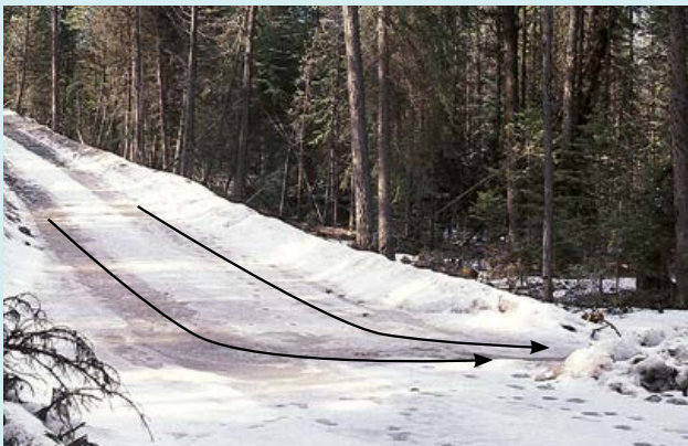
During snowmelt periods, water is directed through the snow berm break.
