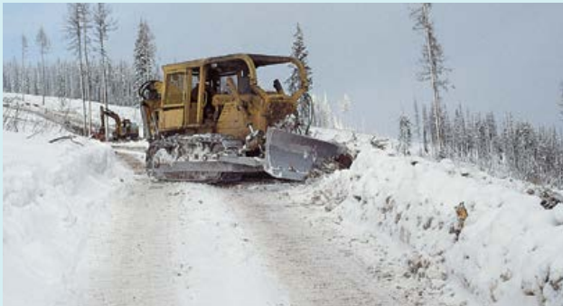
Snow berm breaks allow for drainage during snowmelt without damaging the road surface. They also serve as escape corridors for wildlife.
