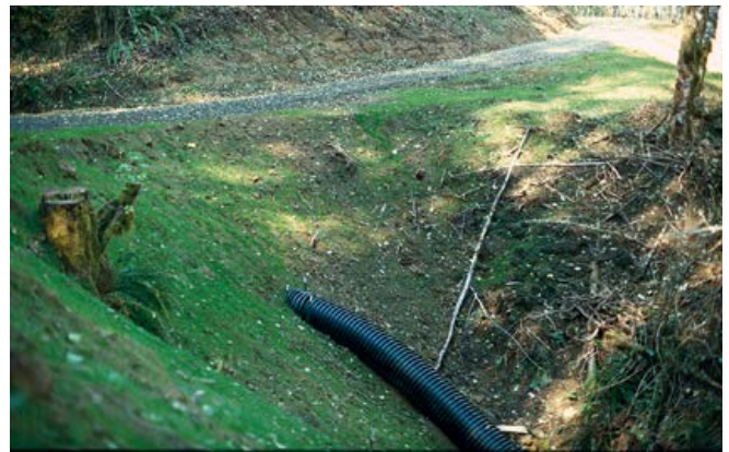
The flexibility of a plastic pipe makes it a popular alternative to a metal culvert.
